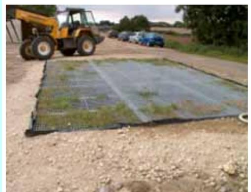
Most pesticide breakdown takes place in the top area of a Lined Biobed so the surface area for absorption/activity is more important than depth. There should be a minimum ratio of 1m<sup>2</sup> surface area per 1m<sup>3</sup> of liquid. As a general rule of thumb, if using the Indirect design, the surface area of the Lined Biobed should be approximately two-thirds of the area from which it is receiving run off.
