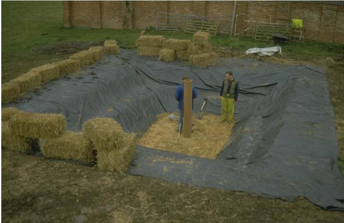
**Plate 1 Field biobed under construction**
