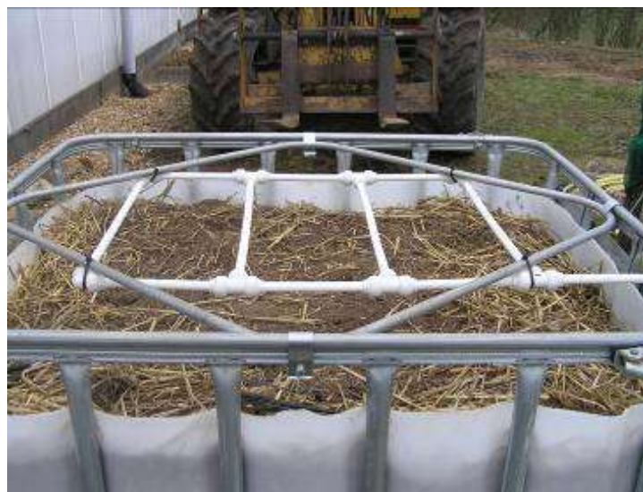
Plate..... Distribution pipe work above each IBC
