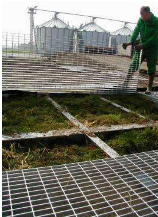
Example of grid construction used to allow access to direct biobed systems
