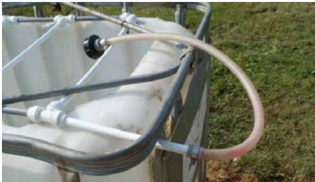
Connect sufficient reinforced hose to join the plastic pipe to the IBC hose tail on two IBC's, secure with a jubilee clip at either end.
