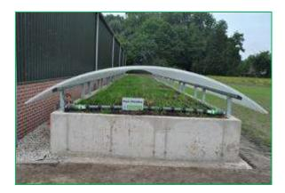
Another system operates in a similar way to the biobed but the biomix is held within a concrete box or trough some 600mm deep, this being covered with a translucent roof above an air gap as before. Again no discharge is intended with this system.
