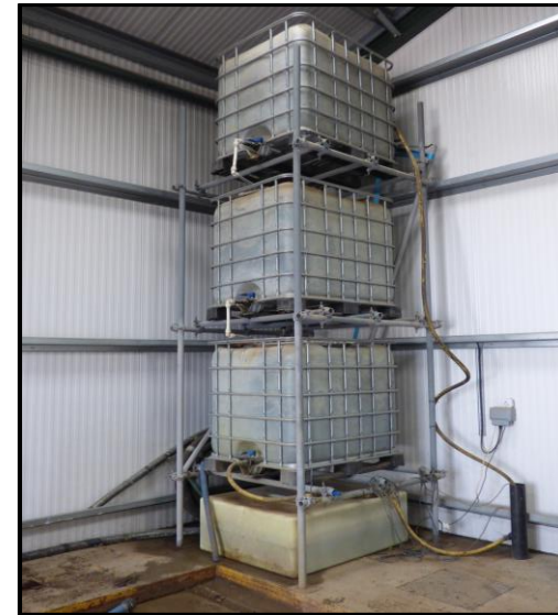
Biofilter showing frame and coupling system including low tank to discharge to external irrigated area or recycle to top to maintain moisture in biomix.
