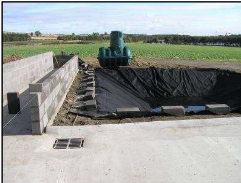
Indirect biobed system under construction. Bunded handling area in foreground, with a boom wash out section all draining to single collector. Background – liner within hole waiting to be filled with biomix and secure intercept tank awaiting installation.
