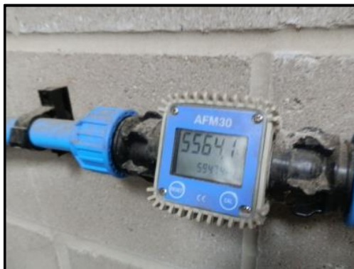
Biofilter in sprayer centre shed, extremely clean operation and flow meter fitted for interests' sake to discharge showing annual use.
