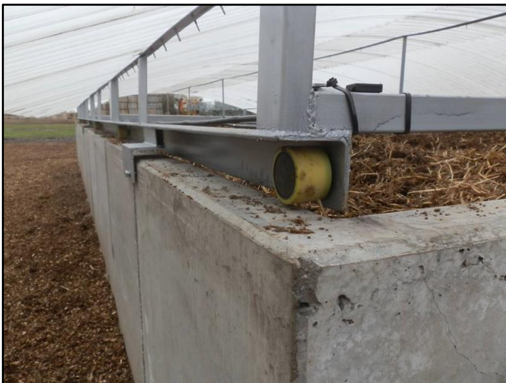
Phytobac installed in Cambridgeshire, concrete panel container. Detail of sliding roof and drip irrigation below.
