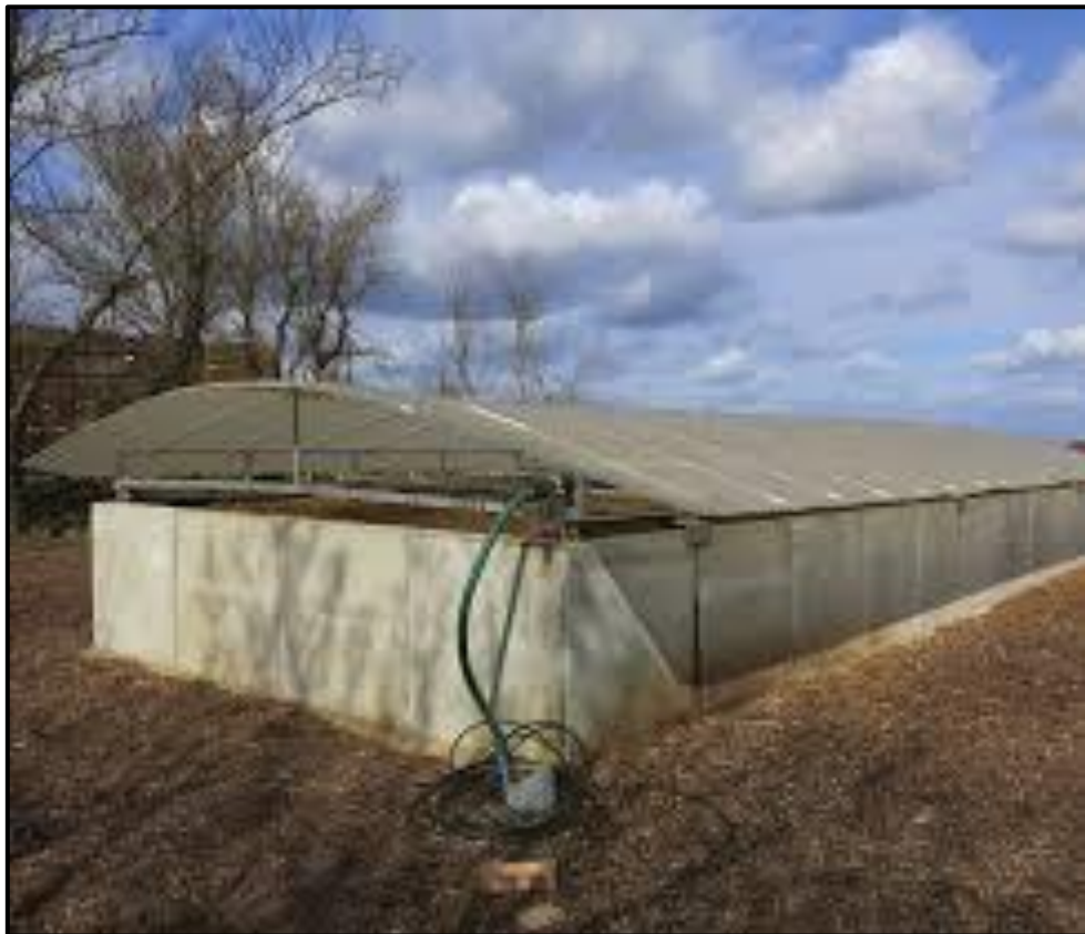
Phytobac installed in Cambridgeshire, concrete panel container. Detail of sliding roof and drip irrigation below.
