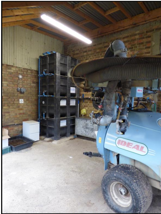
Horticultural fruit spraying operation. Small lean to onto existing sheds, constructed using farm labour incorporates central drain to biofilter.
