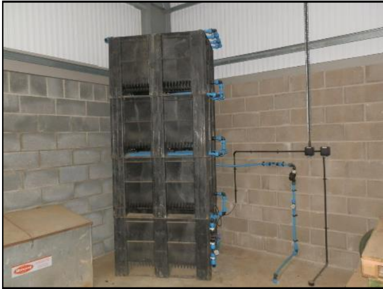
Biofilter in sprayer centre shed, extremely clean operation and flow meter fitted for interests' sake to discharge showing annual use.
